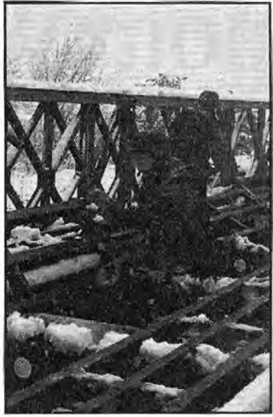
Staff Sgt. Anthony Gloriani lifts part of the bridge decking to put sway bracing underneath to strengthen and keep the Bailey bridge straight.
