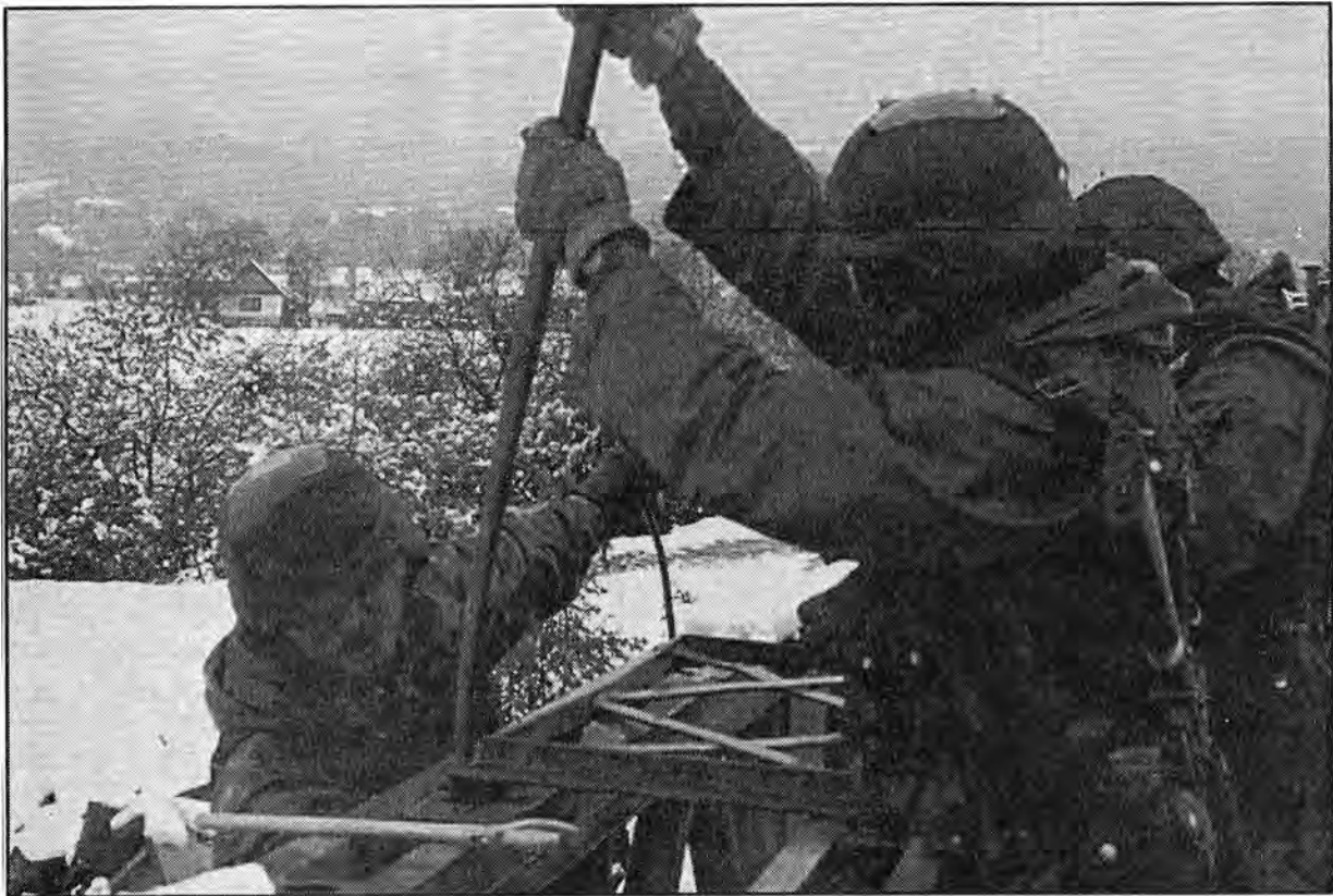
Staff Sgt. Anthony Gloriani and Staff Sgt. Raphael August fit a top bracket onto a Bailey bridge to straighten and strengthen the bridge.
