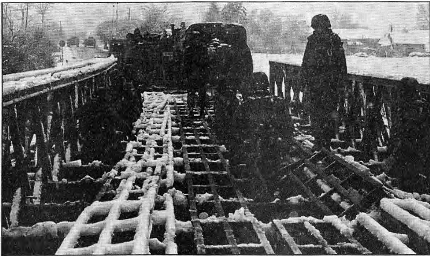
B Company, 82nd Engineers, put new sway bracing under the deck of a Bailey bridge emplaced by the Serbian army after the original bridge was destroyed by a bomb. The bridge became unsafe for heavy vehicles and was repaired by 82nd soldiers during a late April snowstorm.
