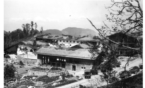
In the area of the hotel, damage from bombing and shelling was obvious.
